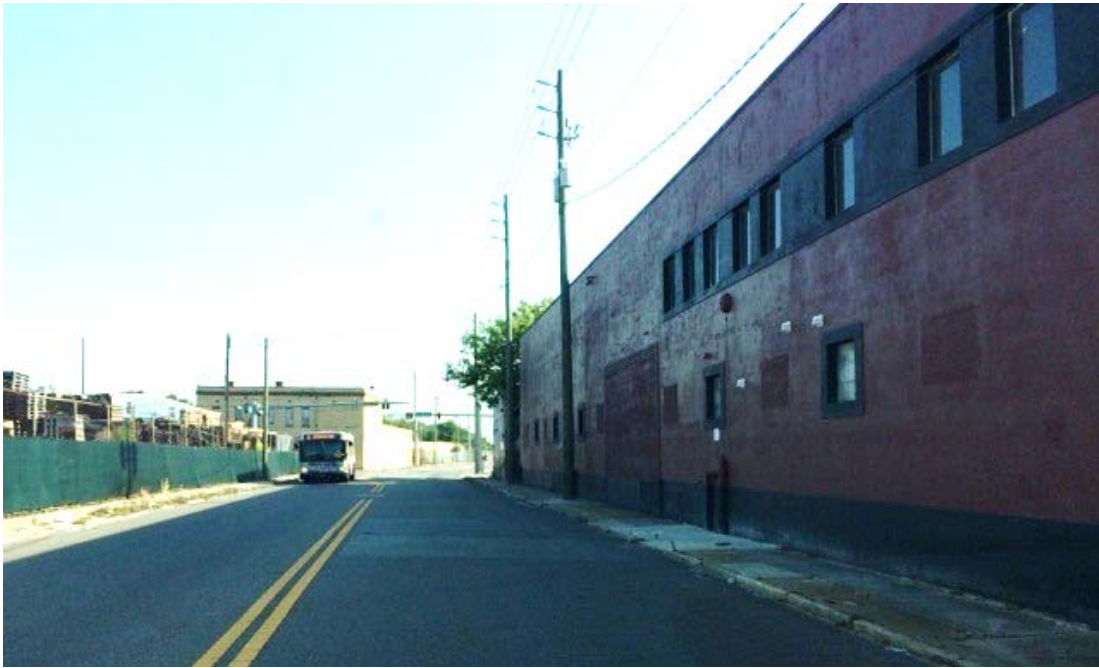
The subject site on the right facing north along Myrtle Ave. towards Beaver St.
