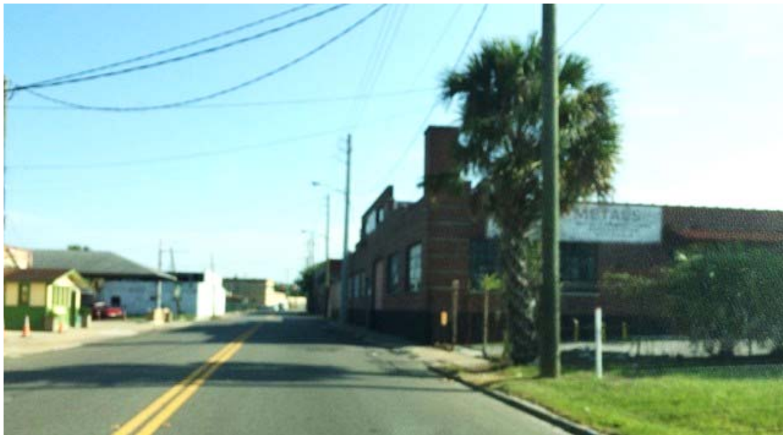
The subject site on the right facing north along Myrtle Ave.
