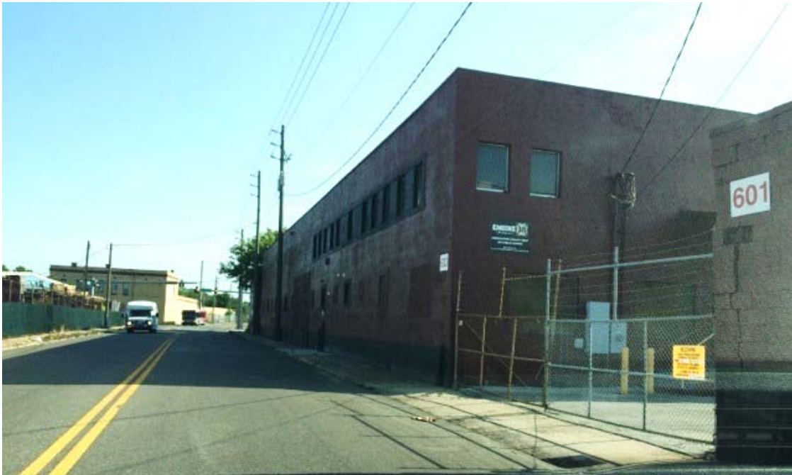
The subject site on the right facing north along Myrtle Ave.
