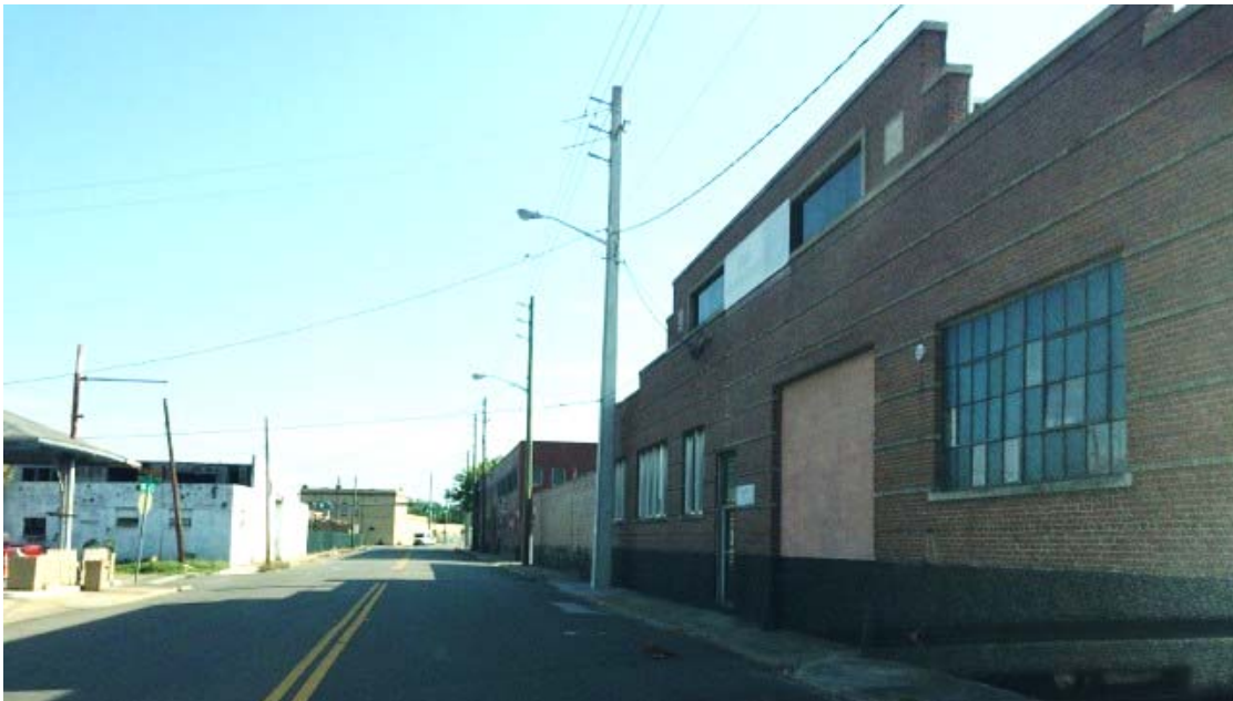
The subject site on the right facing north along Myrtle Ave.
